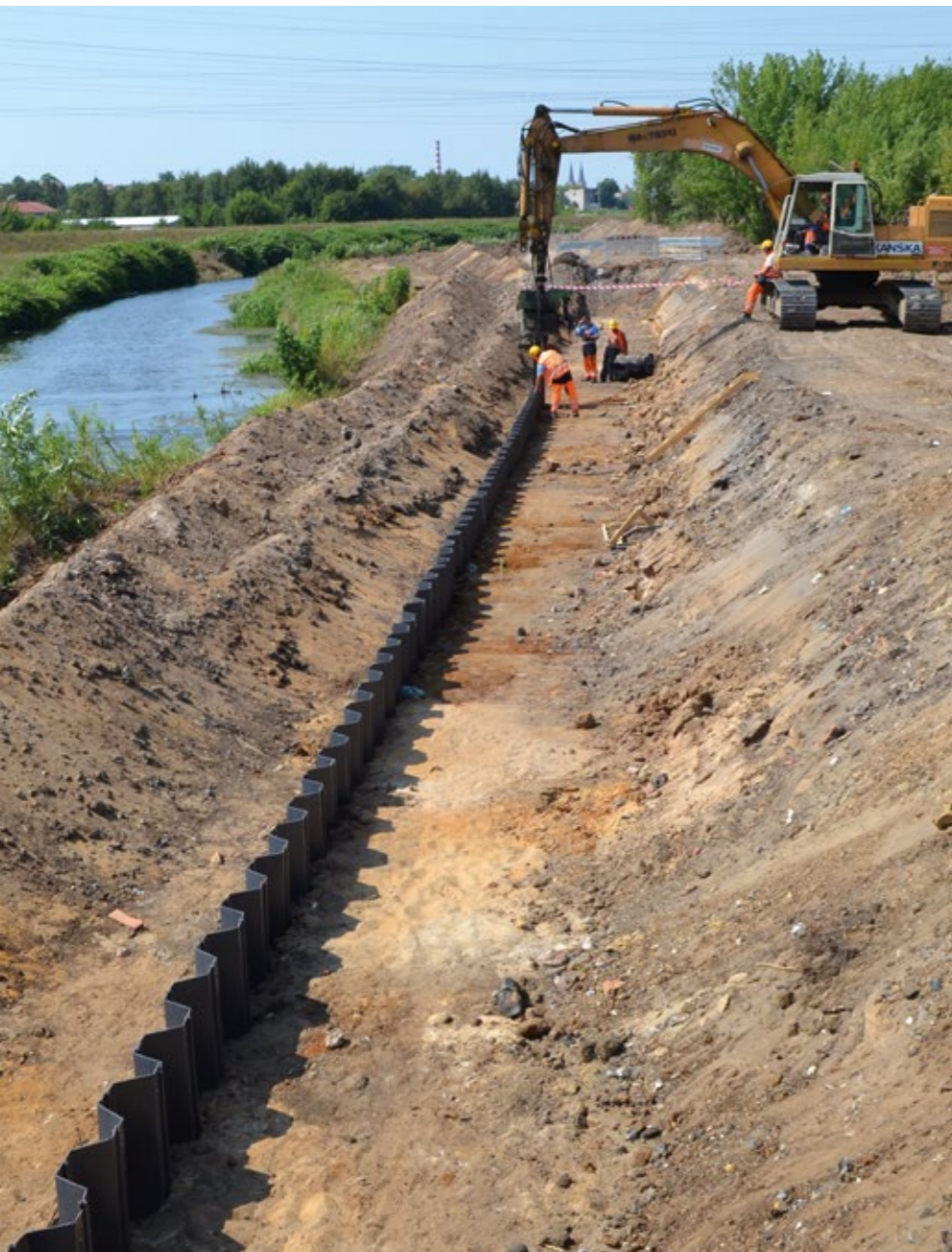
CZĘSTOCHOWA, POLAND: REINFORCEMENT OF A FLOOD EMBANKMENT.
