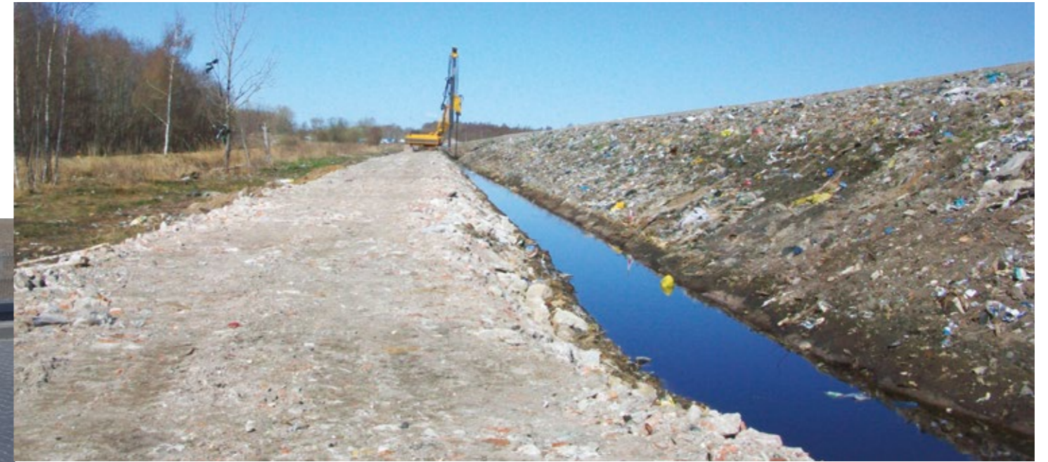
PARNU, ESTONIA: INSTALLATION OF A CUT-OFF WALL AT A TANNING FACILITY CHEMICAL WASTEYARD.
