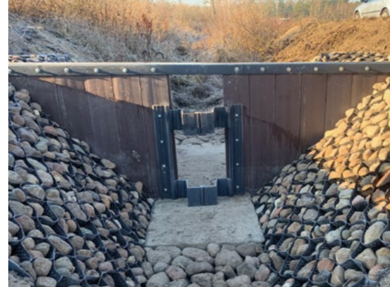
GRABÓW, POLAND: ANOTHER TYPE OF A SMALL RETENTION SLUICE INSTALLED WITHIN ONE DRAINAGE AREA IN THE PILICA RIVER BASIN.
