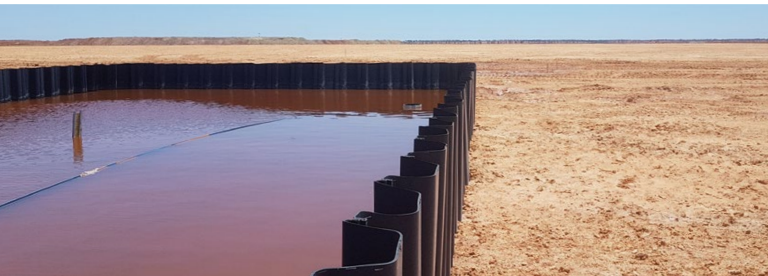
WILUNA, AUSTRALIA: BRINE RESERVOIR CONSTRUCTED USING VINYL SHEET PILES WITH INTEGRATED GASKETS MADE OF SOFT PVC.
