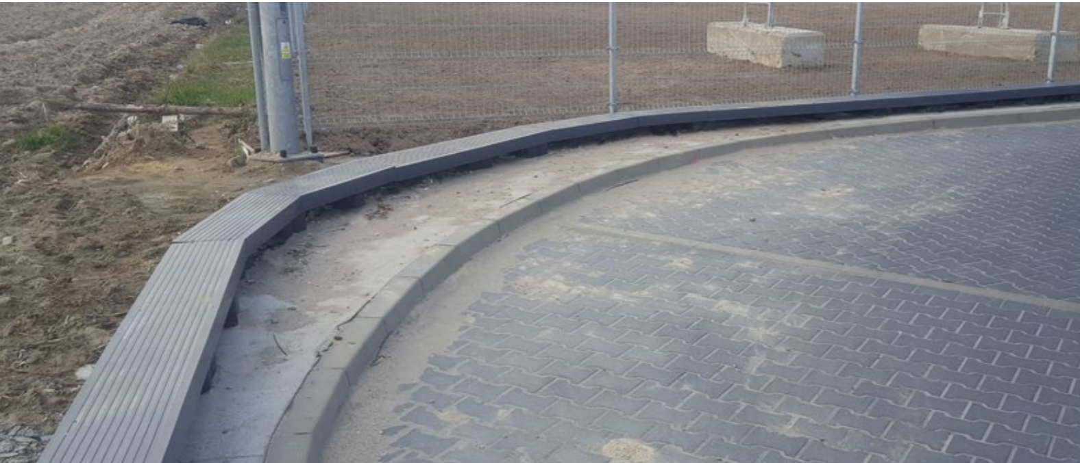
KUTNO, POLAND: PROTECTION OF A PETROL STATION AGAINST FLOODING FROM THE SURROUNDING FIELDS, ENHANCING THE RETENTION CAPACITY OF THE AGRICULTURAL AREA BY REDIRECTING THE WATER FILTRATION ROUTE, AS WELL AS PROTECTING THE ADJACENT FARMING LAND AGAINST POSSIBLE CONTAMINATION WITH CHEMICAL SUBSTANCES.
