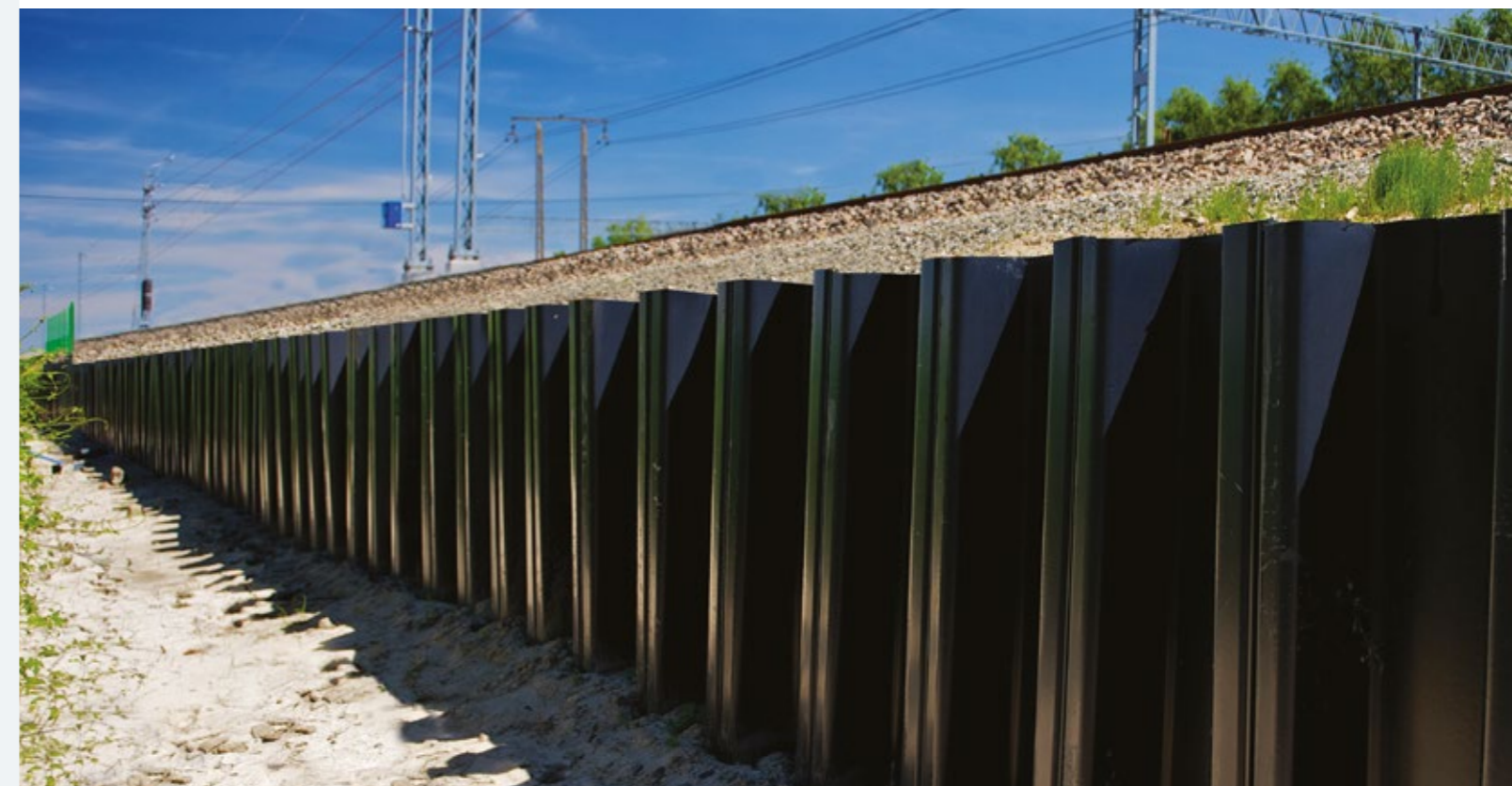
PRUSZKÓW, POLAND: RAILROAD EMBANKMENT STABILIZATION.
