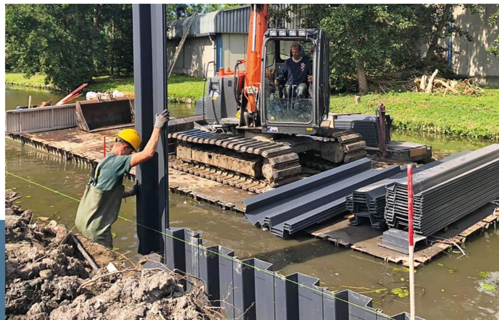
DELFT, THE NETHERLANDS: REINFORCEMENT OF A CANAL EMBANKMENT.
