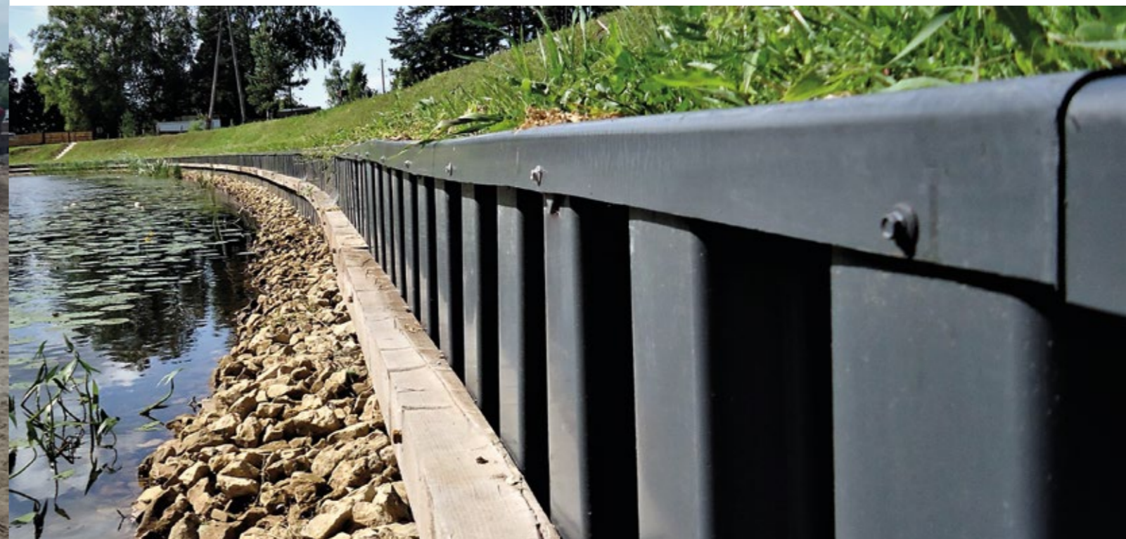
CARNIKAVA, LATVIA: EMBANKMENT REINFORCEMENT OF A WATER RESERVOIR.
