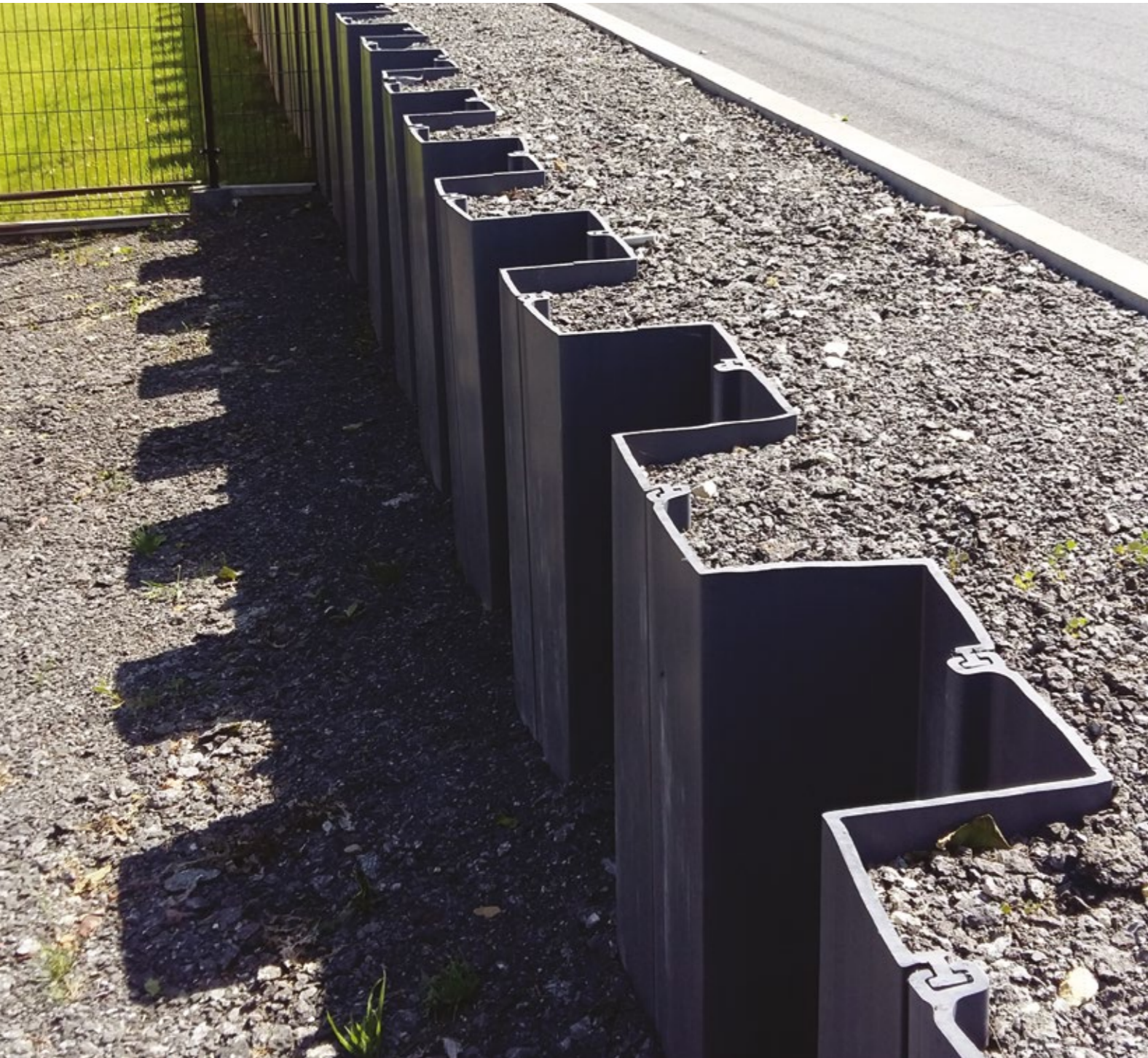
MARKLOWICE, POLAND; RETAINING WALL IN A ROAD CONSTRUCTION.
