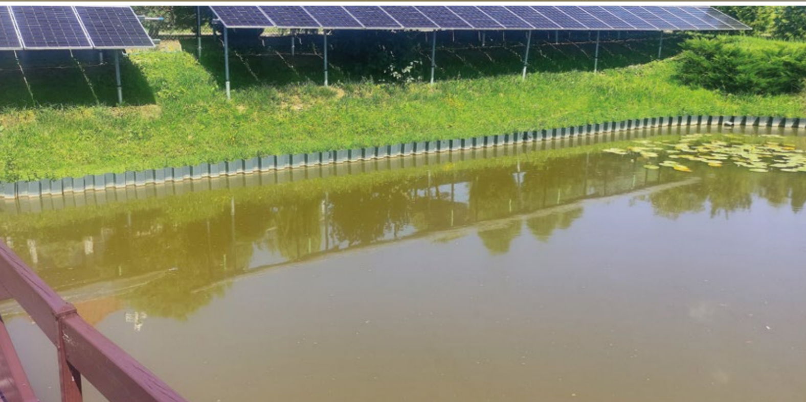
OLECKO, POLAND: VINYL SHEET PILES USED TO REINFORCE AN EMBANKMENT OF A PRIVATE POND.
