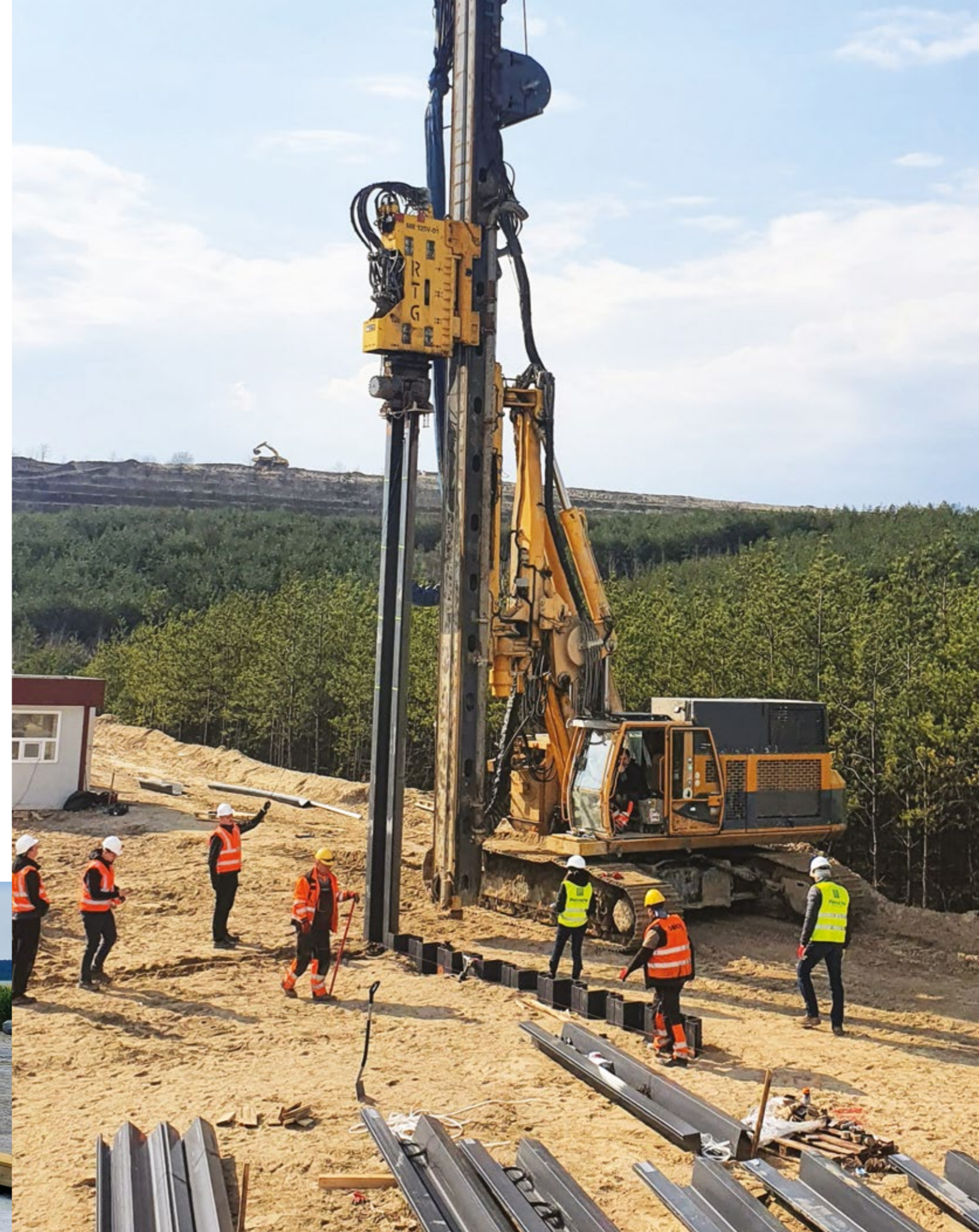
THE OLKUSZ AREA, POLAND: DRIVING OF THE SUPERLOCK HYBRID SHEET PILES IN ADVERSE SOIL CONDITIONS.
