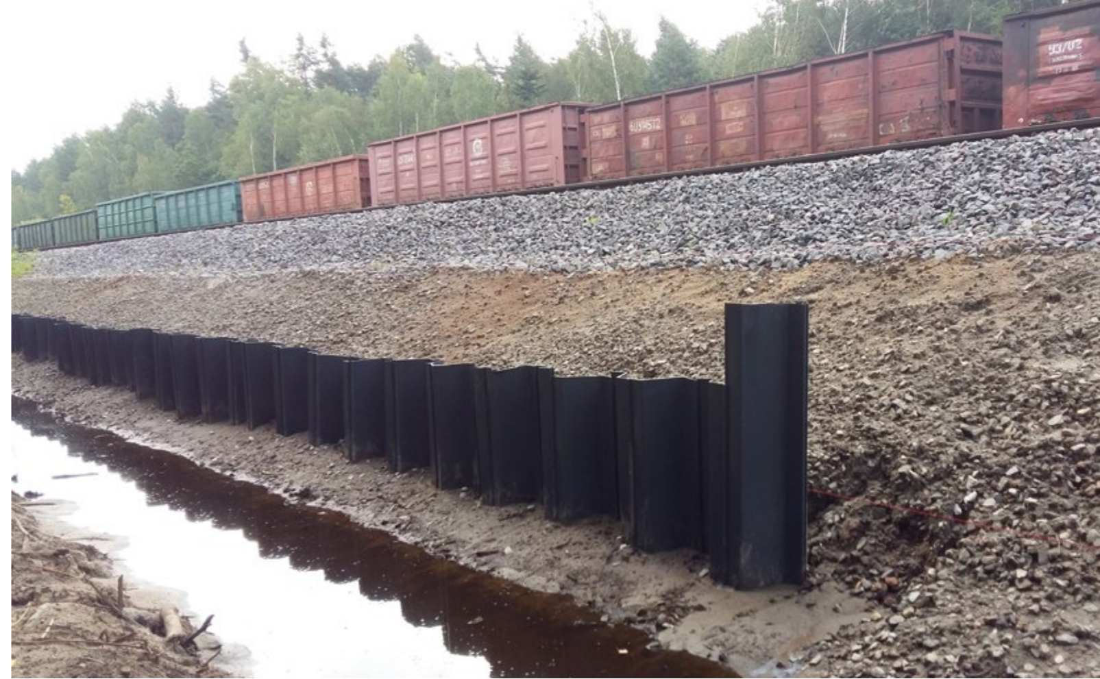
STALOWA WOLA, POLAND: STABILIZATION OF A RAILROAD EMBANKMENT.
