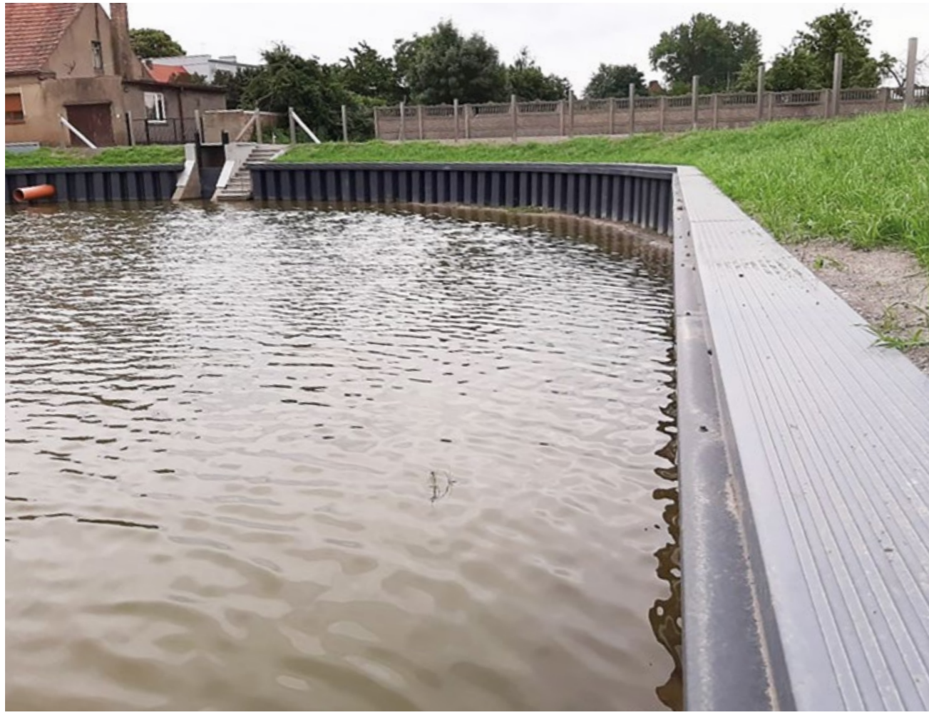
THE POZNAŃ AREA, POLAND: REVITALIZATION OF A WATER RESERVOIR - EMBANKMENT STABILIZATION WITH A VINYL SHEET PILING PALISADE FINISHED WITH A CAP AND MODERNIZATION OF WATER DISCHARGE BY INSTALLATION OF MODULAR VINYL SLUICE IN THE EXISTING WEIR.
