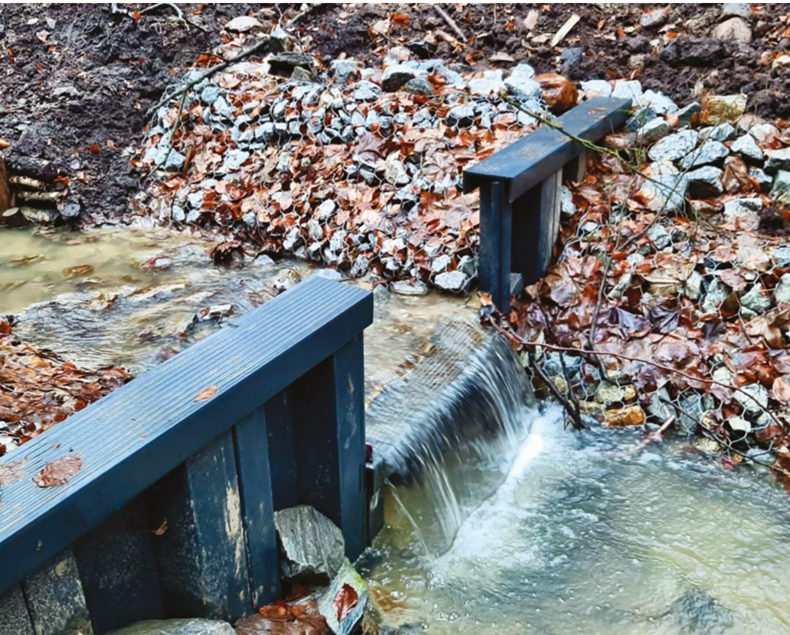
SZCZECIN, POLAND: SYSTEM OF WATER BARS INSTALLED AT A STREAM TO SLOW DOWN WATER RUN-OFF.
