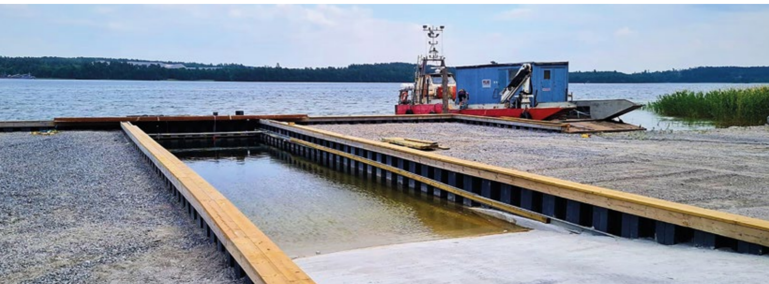
UPPSALA, SWEDEN: HYBRID SHEET PILES USED TO CONSTRUCT A BOAT RAMP.
