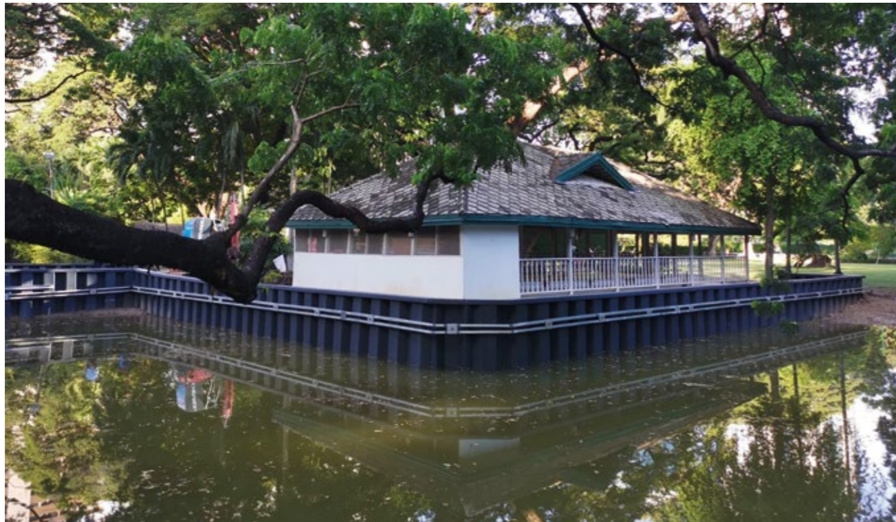
BANGKOK, THAILAND: VINYL SHEET PILES USED TO DEVELOP BLUE INFRASTRUCTURE AT THE US EMBASSY.
