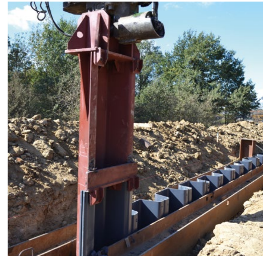
THE WROCLAW WATER JUNCTION, POLAND: REINFORCEMENT OF A FLOOD BANK WITH VINYL SHEET PILES - INSTALLATION WORKS.
