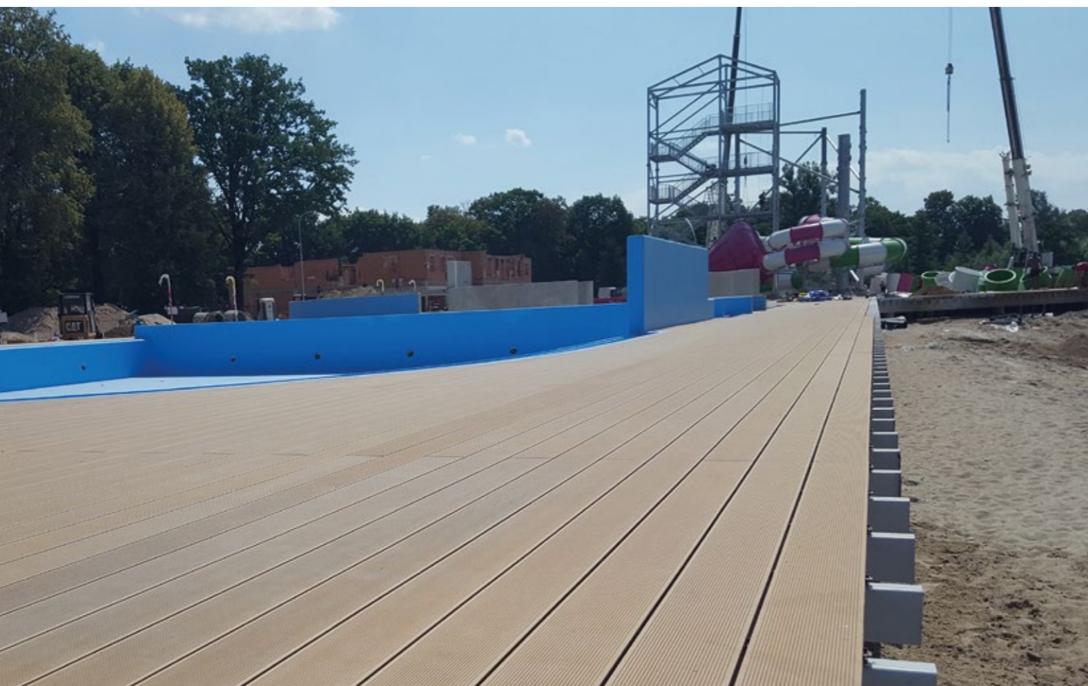
IN THIS PROJECT, APART FROM THE ECOLOCK VINYL SHEET PILING, THE TERRADECK COMPOSITE PLANKS WERE USED.
