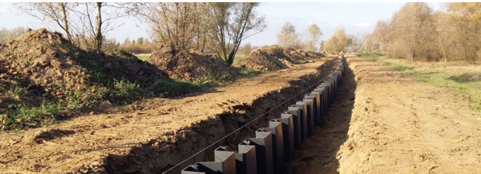
GIZAŁKI, POLAND: REINFORCEMENT OF FLOOD EMBANKMENT.
